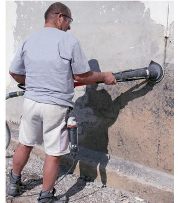
Grinding bitumen coating with PCD grinding disc
