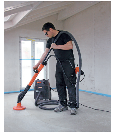
Grinding screeds
