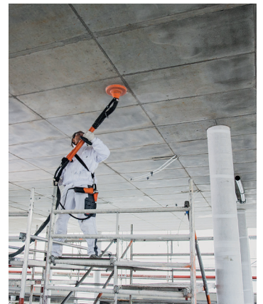
Grinding fair-faced concrete
