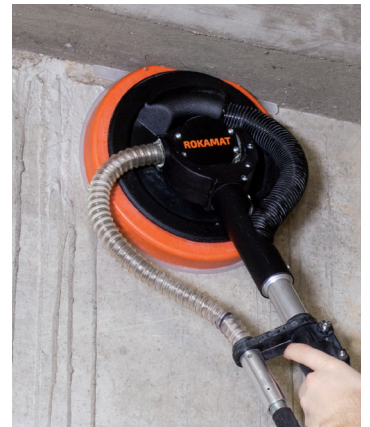
Grinding concrete burrs
